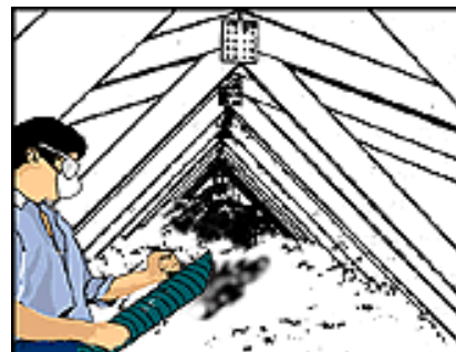
Blown-in attic insulation
